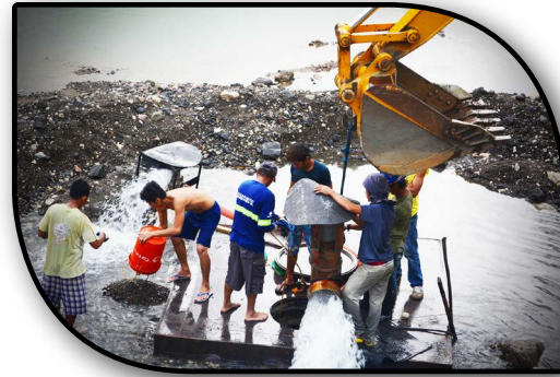
Manual declogging at Manhole No. 4 to restore the operation of the Infiltration Gallery. A pump was used in dewatering the manhole, which was necessary for the removal of stones and pebbles.
