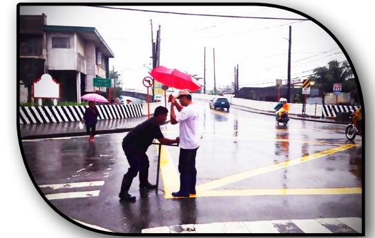
Valve rationing conducted by flushing personnel near Magsaysay Bridge.
