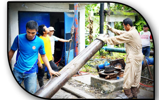
Rehabilitation activities, i.e., installation of pump/motor, and pipes, for the reactivation of Pump Station No. 10.
