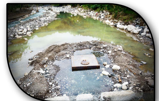
The new cover of Manhole No. 4
