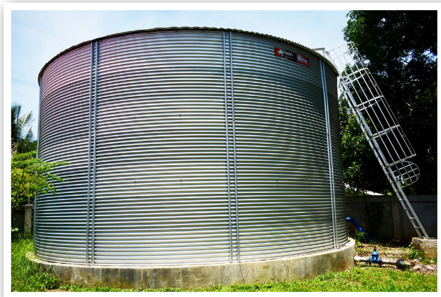
Pinamanculan Ground Tank
