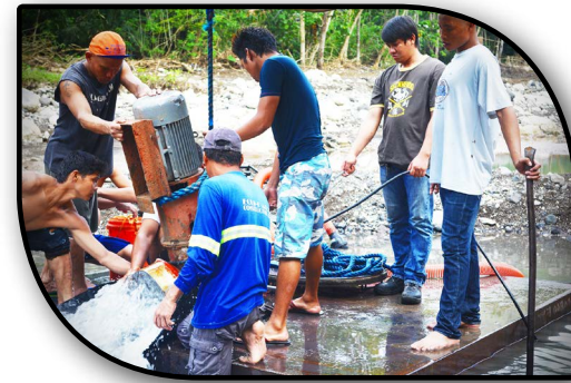
Declogging activity at Manhole No. 4 with the aid of pumping equipment.
