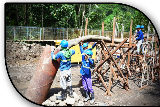
An 8-inch flexible hose serving as discharge line of the centrifugal pumps directed to the 600-mm interconnection pipe.
